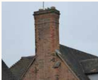
Queen Anne chimney
