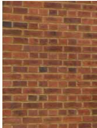
English bond brickwork
