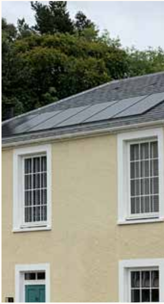
Flush Solar PV panel
