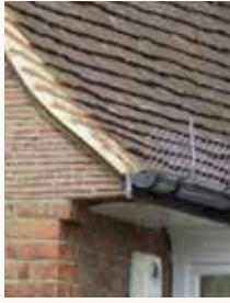
Sprocketed eaves detail
