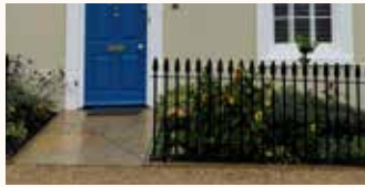
Ramp to dwelling
