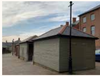
Timber-clad bin store
