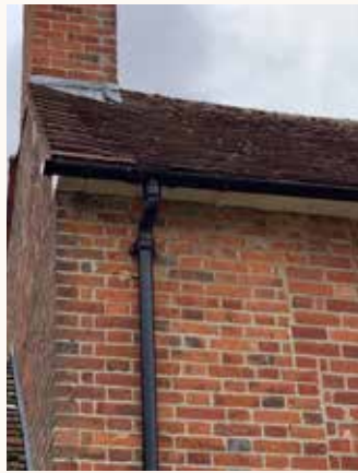
Painted metal rainwater goods
