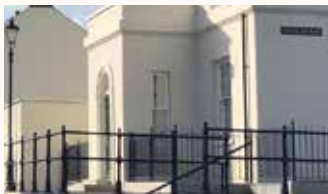
Formal enclosed porch
