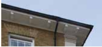
Projecting eaves with brackets
