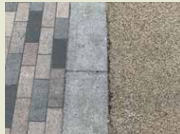
Flush conservation kerb
