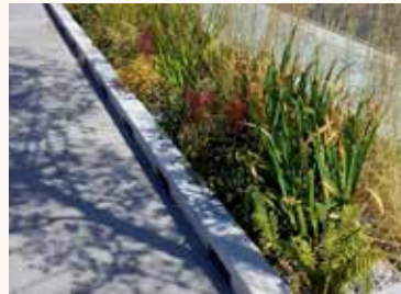
Kerb channel drain to swale system
