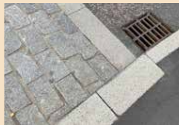
Granite sets in contrasting colour (example uses include drainage areas in verges and at junctions)
