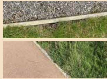
Timber edge (above) Concrete 50mm kerb (below)
