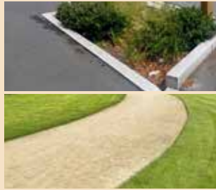
Asphalt (above) Breedon gravel (below) Surfaced dressed gravel
