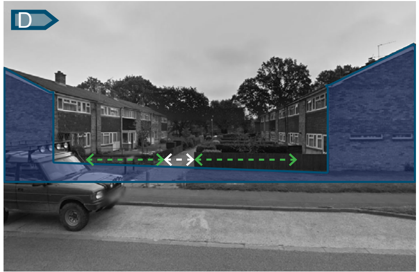
Area 7: Blaven Walk, looking east at Barnfield Court.
