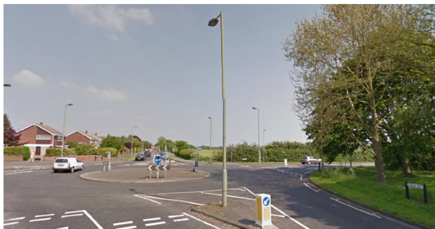
FIGURE: 24 EXISTING HIGHWAYS
