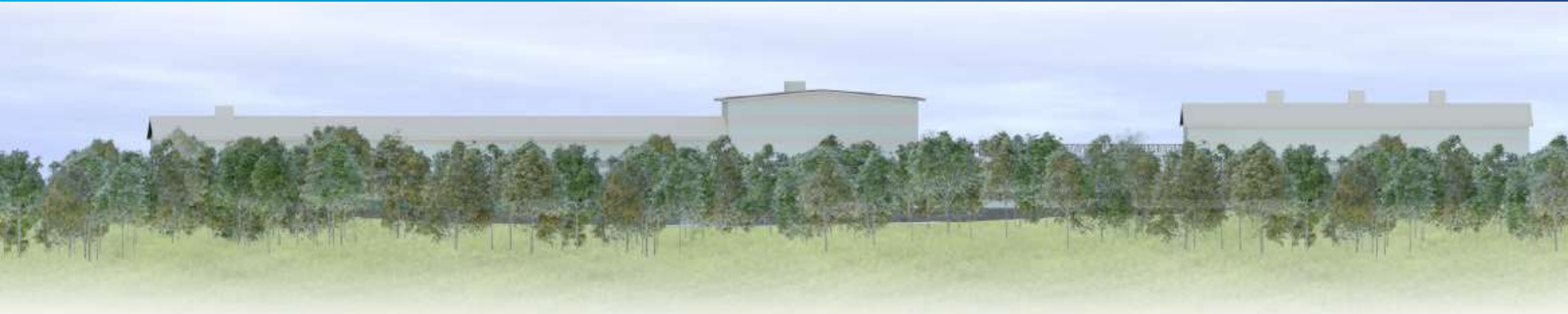
Showing mitigation planting and mounding in future open space (at Daedalus North) in conjunction with the Converter Station buildings
