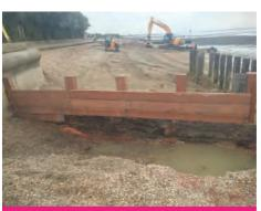
Phase 1 of the Hill Head project is now complete. New shingle has been laid and groynes have been rebuilt to help protect the promenade from wave damage.
