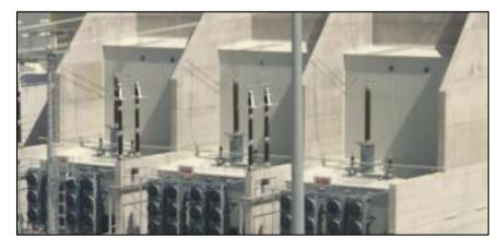
Figure 3 - Example of power transformer contained by audible noise enclosure
